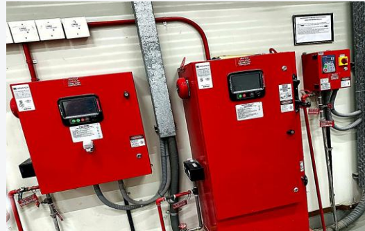
Fire Pump Controller Panels Diesel, electric, and jockey pump controllers
