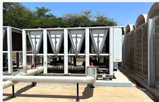
Chiller Units — Perimeter Screen Wall Chiller installation along the plant perimeter
